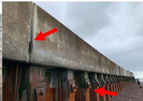
57776 Loss of paint system and surface corrosion of toe piles. Loss of majority expansion joint sealant.
