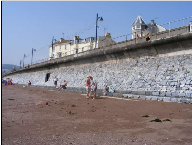
Figure 2.13 Rock-faced, concrete seawall constructed in the mid 1970's.
