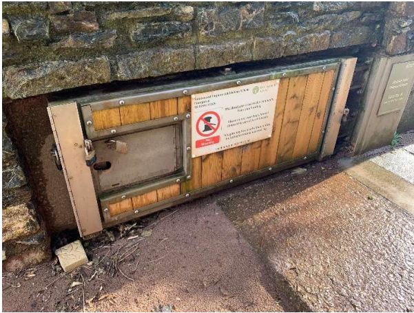
332934 Timber facings to all gates in good condition, no evidence of rot.
