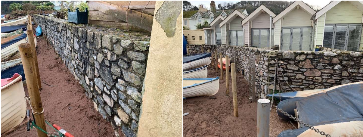
82711 Masonry blocks in good condition, no cracking or gaps in mortar joints, all flap valves present and working. 82719 Masonry blocks in good condition, no cracking or gaps in mortar joints, all flap valves present.
