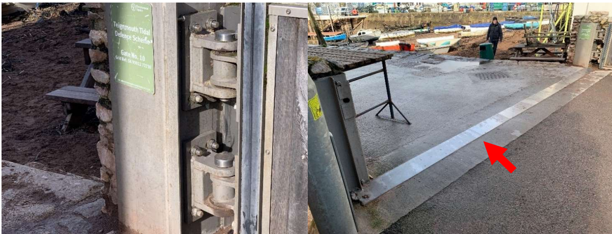
392735 No corrosion to hinges which appear to be in good working order.
