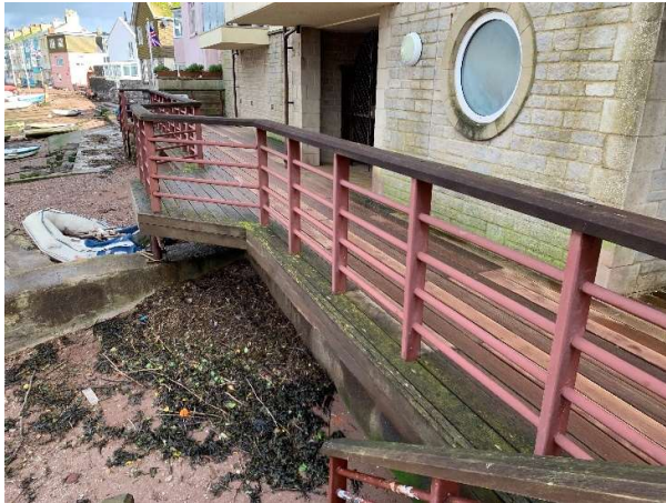
3934 No gaps or damage to timber boards or hand railings along crest of concrete wall.
