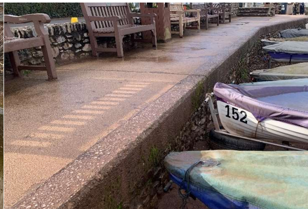
84537 High beach levels along promenade, concrete surfacing and masonry setback wall in good condition.
