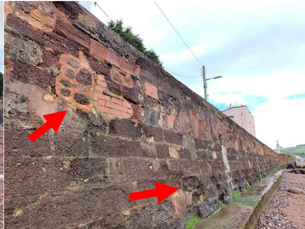
84538 Heavy abrasion to masonry blocks along some sections of wall, especially at toe, many brickwork repairs but in reasonable condition.
