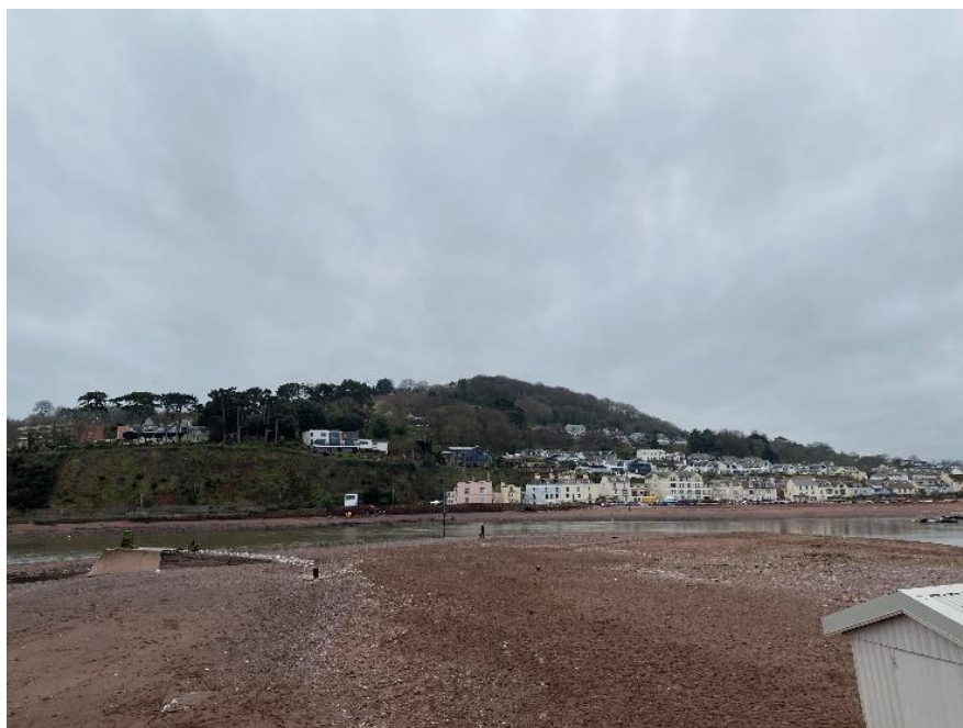
Figure 2-1 Image showing location of The Point breakwater.
