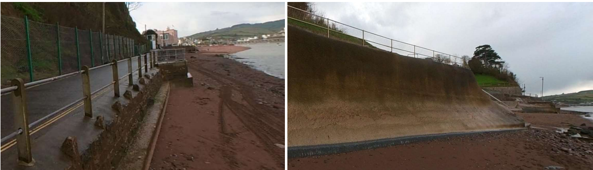
Figure 2.18 Two different seawall types found at Shaldon.
