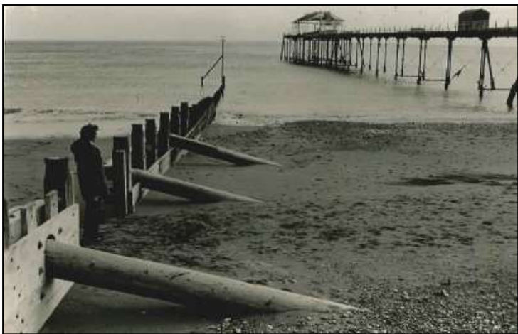
Figure 2.4 Groyne 11, with elevated beach level, in November 1974 (Gundry, 1982).
