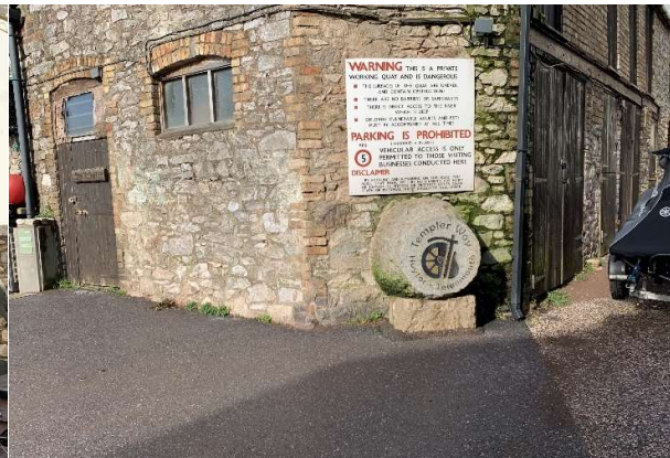
4142 Flood defence alignment appears to run through the Garstone Garden Ornaments property. Not inspected.
