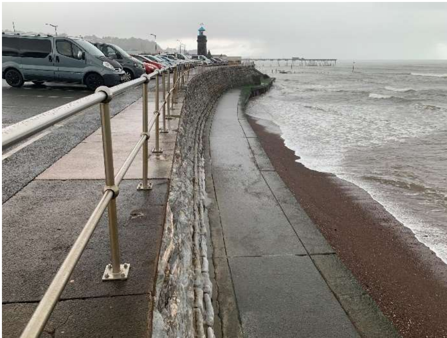
Figure 2.10 Image of the Seawall near The Point Car Park.
