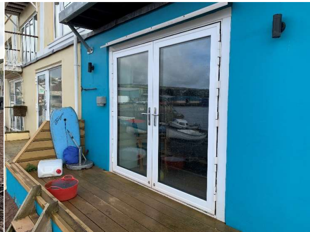
42304 All flood proof doors to property defence line along back of beach in good condition.
