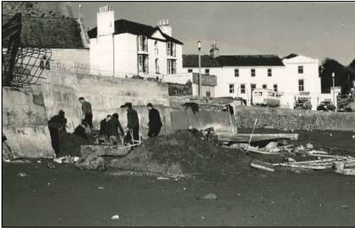
Figure 2.3 Flood defences under construction at Denn Promenade, November 1972 (Gundry, 1982).
