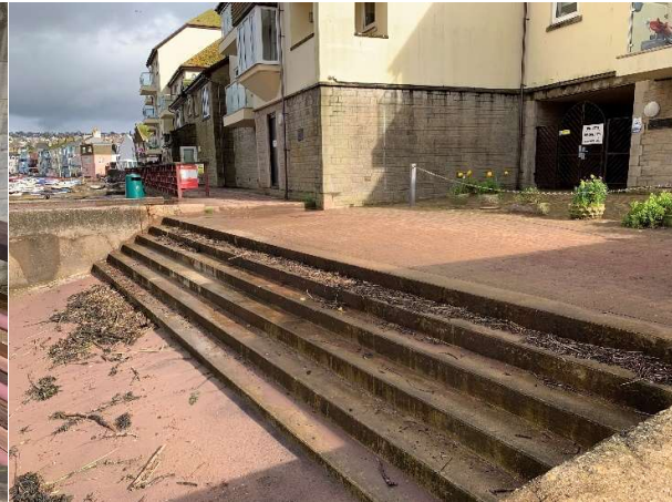
3934 Concrete quay and steps fronting Morgans Quay properties with low levels doors and openings through properties.
